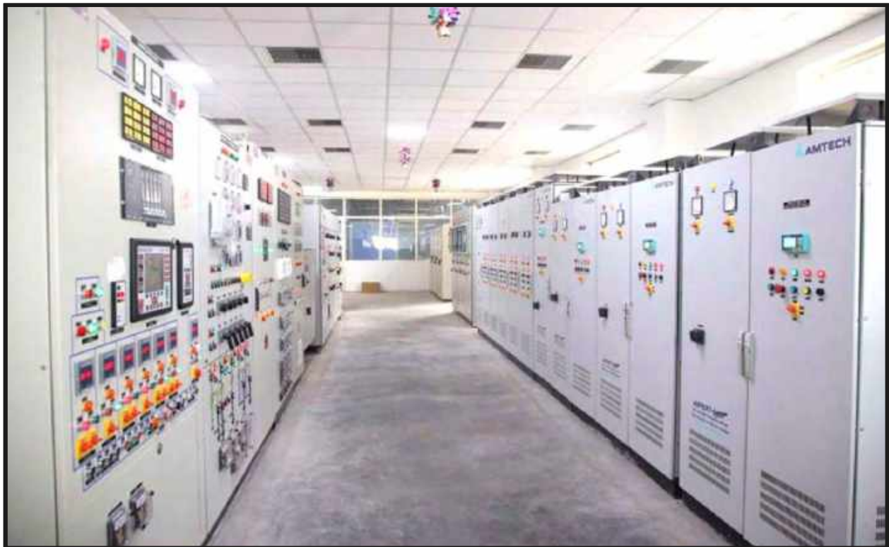
NEW MAIZE PROCESSING FACILITY COMMISSIONED IN PUNJAB
